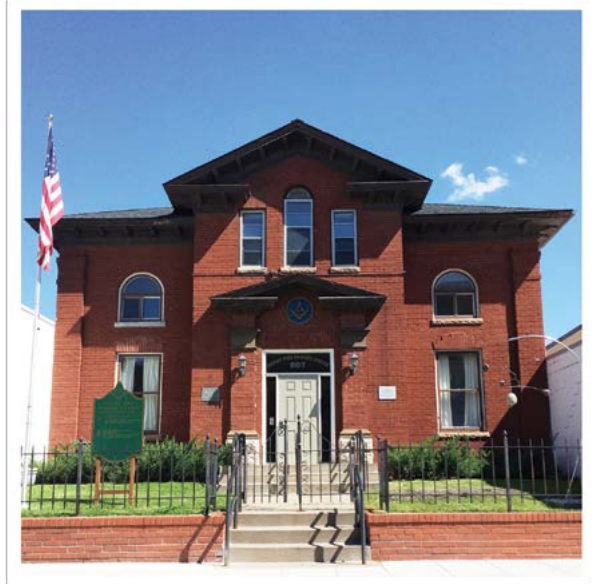
The former Albert Pike Masonic Lodge building will be the future home of the Hopkins History Center.
